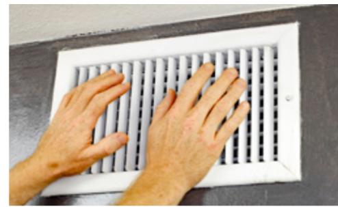
Closing supply vents in unused rooms increases pressure inside ductwork, causing inefficiency similar to a dirty air filter.
